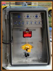
Engraved and paint filled labels are robust and provide a permanence that can withstand wear and tear.
